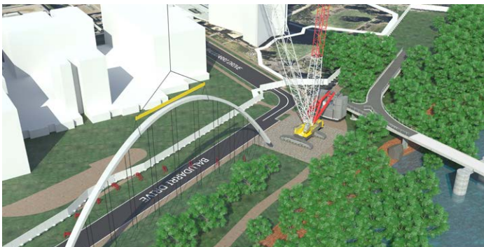
Alfred Street Bridge is an iconic diagonal arch pedestrian bridge supporting eco-friendly city accessibility in Parramatta, New South Wales, Australia.
